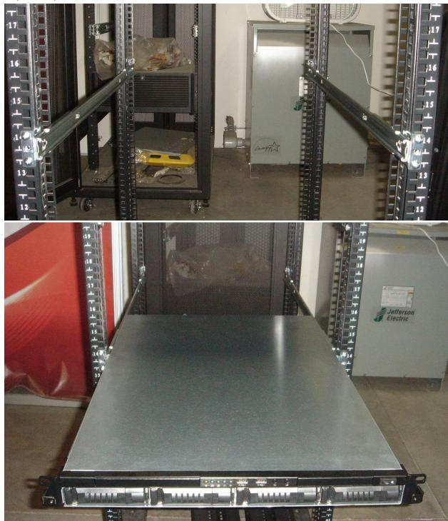
5. Repeat step 4 to mount two rails onto the rack and insert the chassis to the frame.
