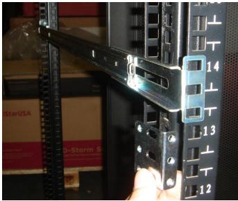
b. Align the mounting bracket to the inside of the mounting square.
