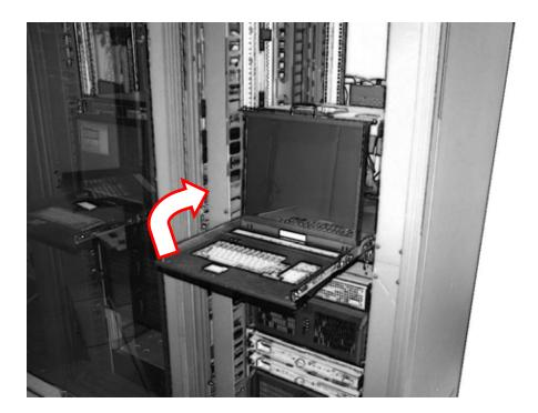
2.9 To turn on the power for the LCD panel, the power button located beneath the LCD can be use to independently turn on/off. LCD screen adjustment button is also located here.
