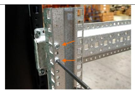
5. Secure both horizontal bars and mounting posts
